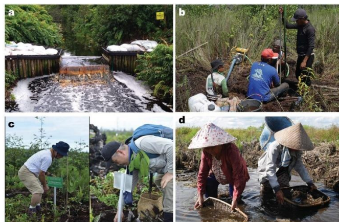
Figure 1. Examples of a) canal block; b) Deep well construction; c) Revegetation; and d) peatland fisheries revitalisation. Source: BRG
